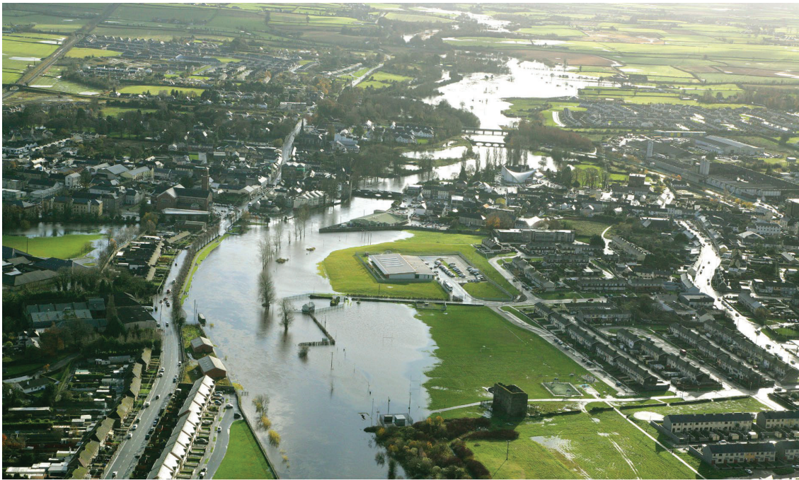
Figure 10.1: Flooding Event Along the River Barrow Floodplain in Athy 2009
