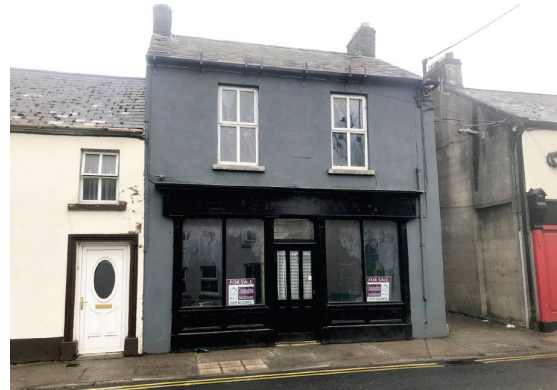
Figure 2.27: Refurbished unit on Offaly St. (July 2020)
