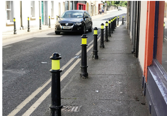
Figure 2.31: Excessive bollards on Offaly Row
