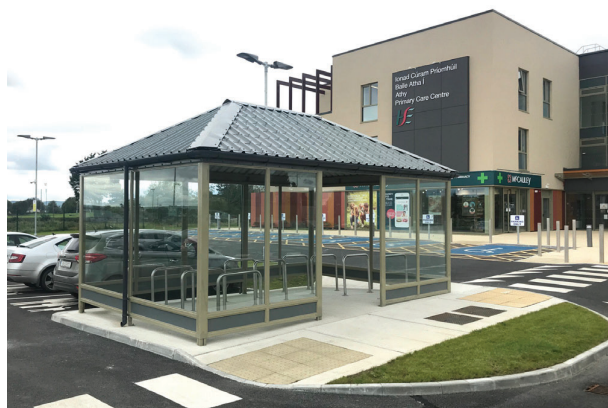
Figure 2.41: Cycling facilities at Athy Primary Care Centre
