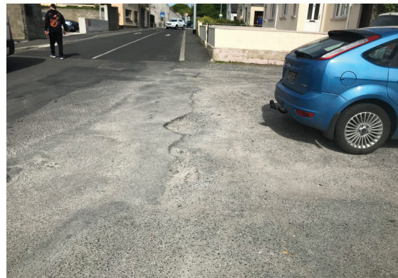
Figure 2.36: Lack of footpath on Meeting Lane
