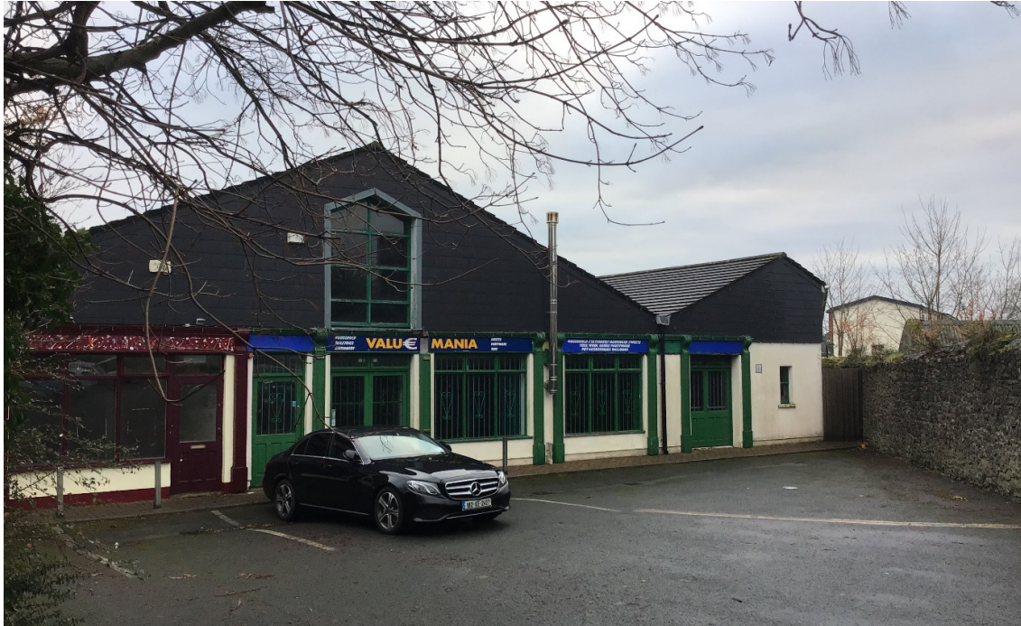
Fig6. Existing Elevation of Units 8 and 9, The Village Centre, Main Street, Clane, Co.Kildare
